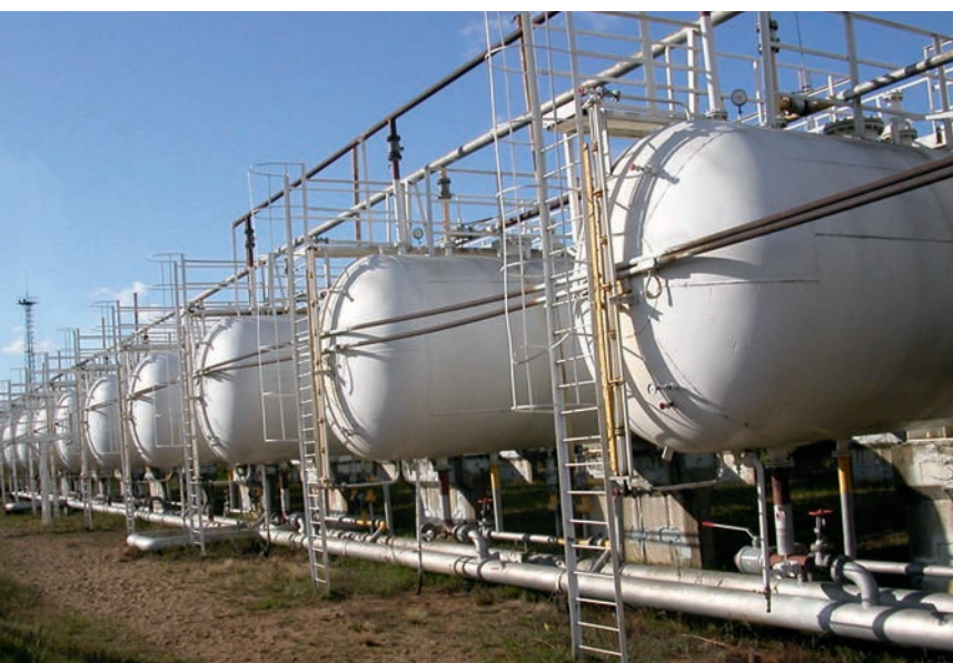
Fig. 3: Liquefied gas tanks, each with a fill capacity of 175 m 3 in Olaine / Latvia. Here, liquefied gas pumps are used.
